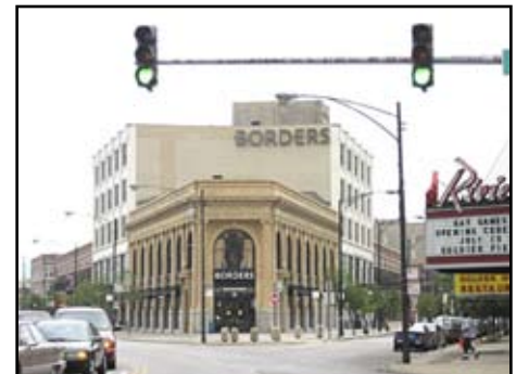
Completed Uptown Square - Lawrence and Racine Joseph Freed's completed Uptown Square redevelopment in 2006
